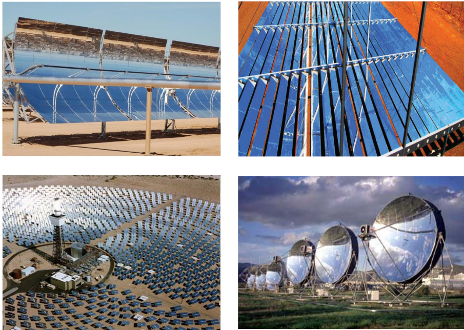
The four types of CSP Technologies: Parabolic Troughs, Fresnel Systems, Central Receivers, and Parabolic Dishes
